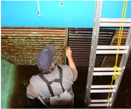
Lang Tank Inspection
